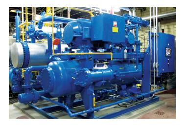
With the lower 60°F (15.6°C) incoming cold water temperature during winter, the estimated heating capacity of the heat pump during winter conditions was estimated at 5.738 MMBtuh (1,682 kW), providing 135 GPM (30.7 m3/h) of continuous 145°F (62.8°C) hot water flow. The heat pump was estimated to provide an average year-round heating capacity of 7.013 MMBtuh (2,056 kW), heating 170 GPM (38.6 m3/h) from 62.5°F (16.9°C) to 145°F (62.8°C).
