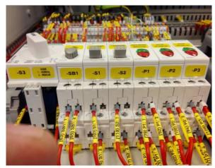
Figure 20: Rescue mode - Control panel front and bottom views
