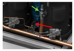
Figure 34: Oil charging service ports
